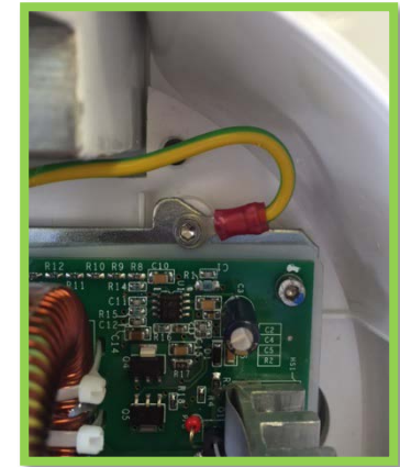
Ground wire #2 from plate bracket
