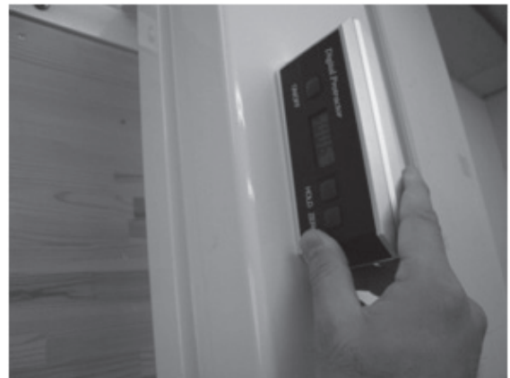
Fig. ③ -31: Checking for column lean (front)
