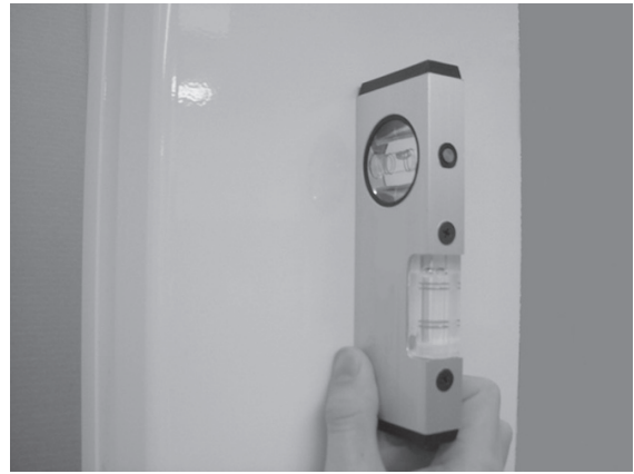
Fig. ③ -26: Checking for column lean
