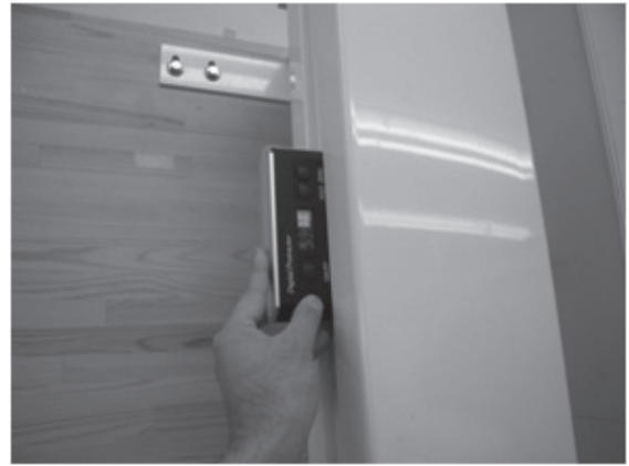
Fig. ③ -30: Checking for column lean (sides)
